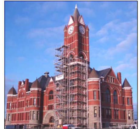
Photo by Gordon Ramstrom, Public Works Architectural Projects Planner
